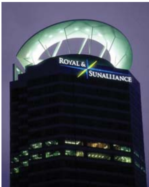
The Royal and SunAlliance building which won an international award for energy efficiency, is a Directenz customer.
